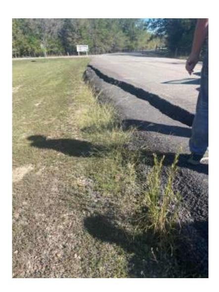
**Paving -** The roadway in the park is in a severe state of disrepair. It was observed that road conditions have degraded from OTRD's original visit in February 2023.
