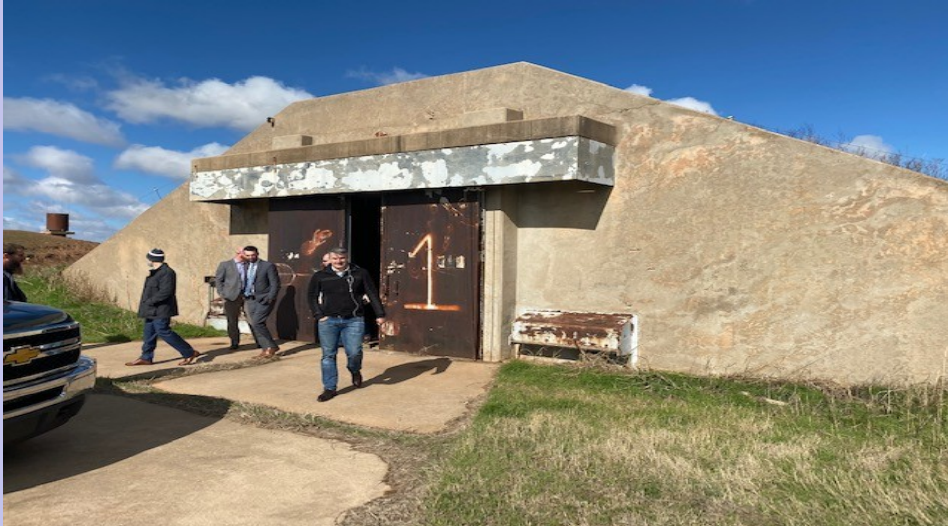
Each 2,000sf bunker has 3' thick walls with 2" steel doors
