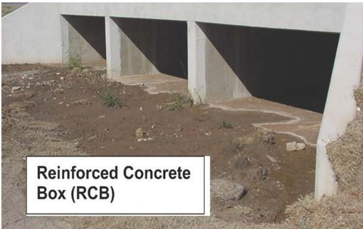
**Reinforced Concrete Box (RCB)**
