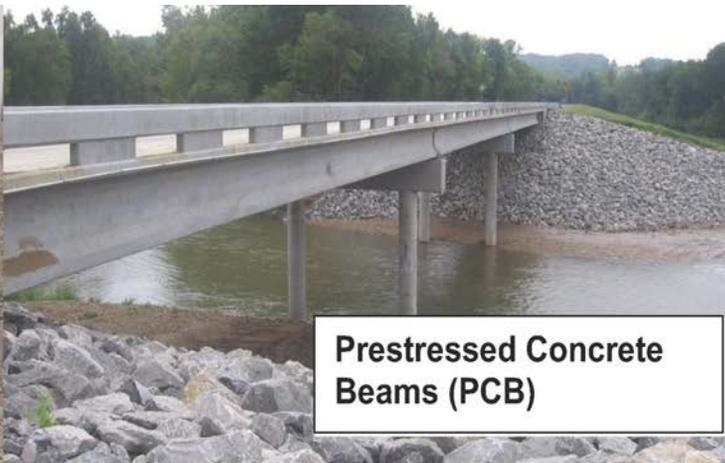
**Prestressed Concrete Beams (PCB)**
