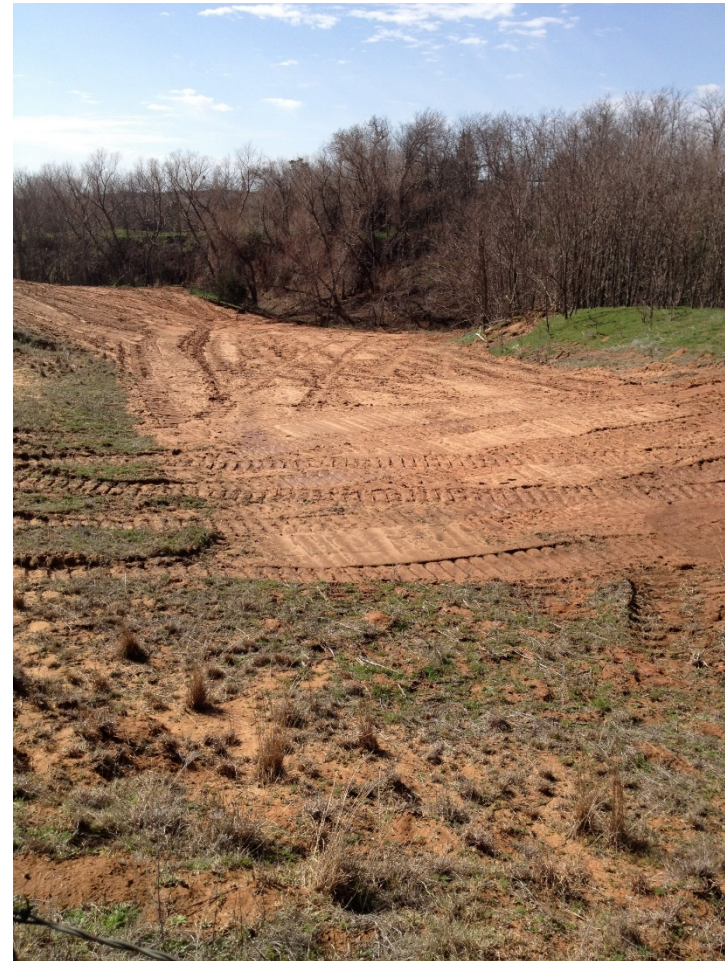
Cowden Laterals 5 - Kiowa County
