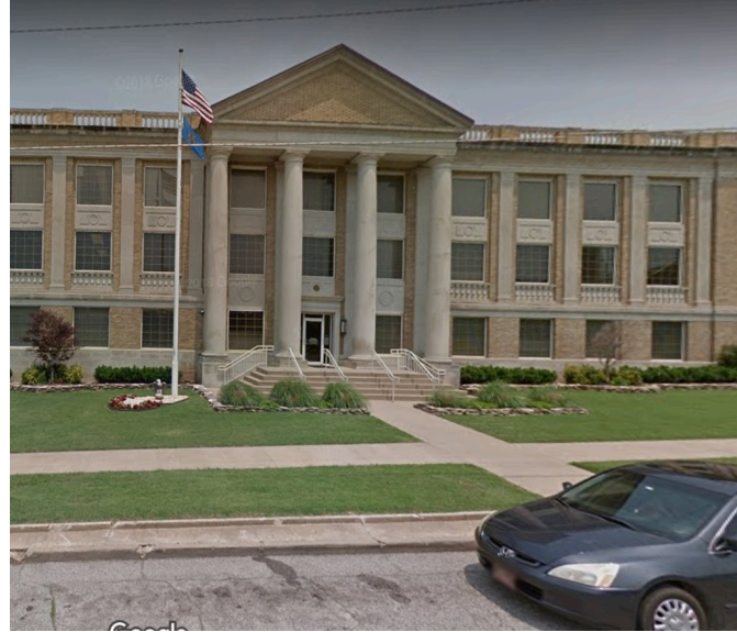
Government Public Meetings on 2 nd floor no accessible route.
