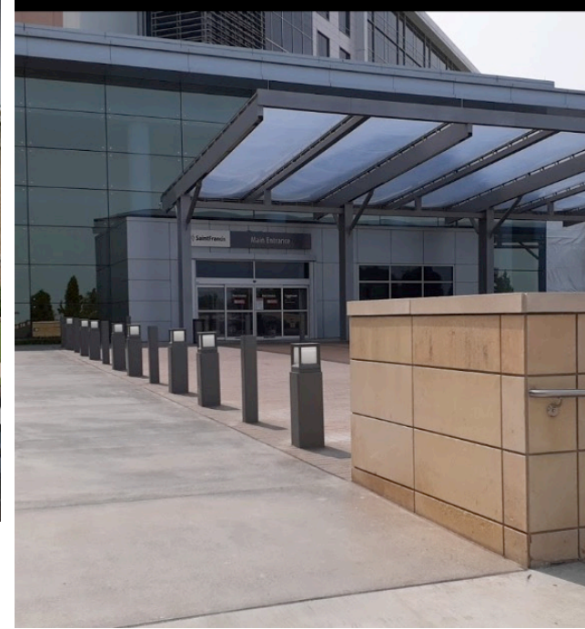
Primary Hospital entrance was a revolving door.
